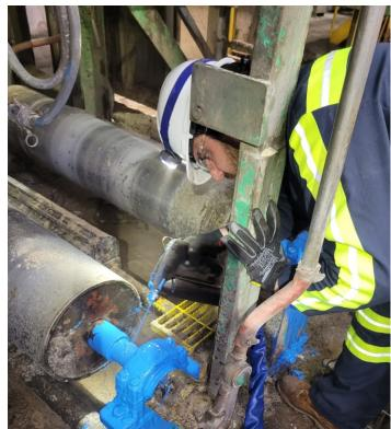
Above, an engineer is shown applying Enviropeel along the bearing shaft. The shaft can freely rotate within the Enviropeel coating which prevents the ingress of contamination.
