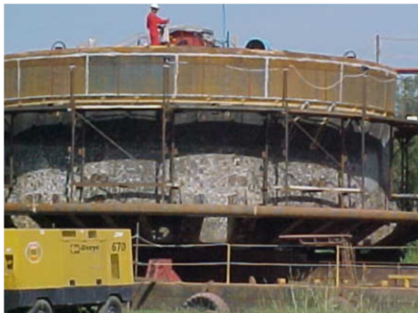
Before and after: left, the main buoy during preparation before coating. Above, after the coating works are complete.
