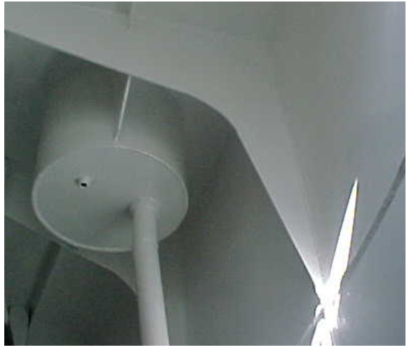
Above: Inside the coffer dams after coating Above left: Buoy bottom after water-jetting Left: Stripe coating cofferdam with 28.15
