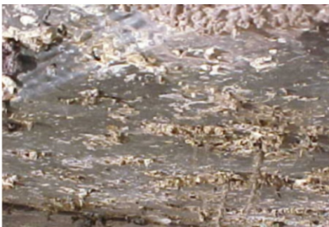
Above: Water-jetting is a fast and clean surface preparation method. Using blast media with the water gave profile, the ability to use Alocit immediately after cleaning while still wet achieved significant cost savings.
